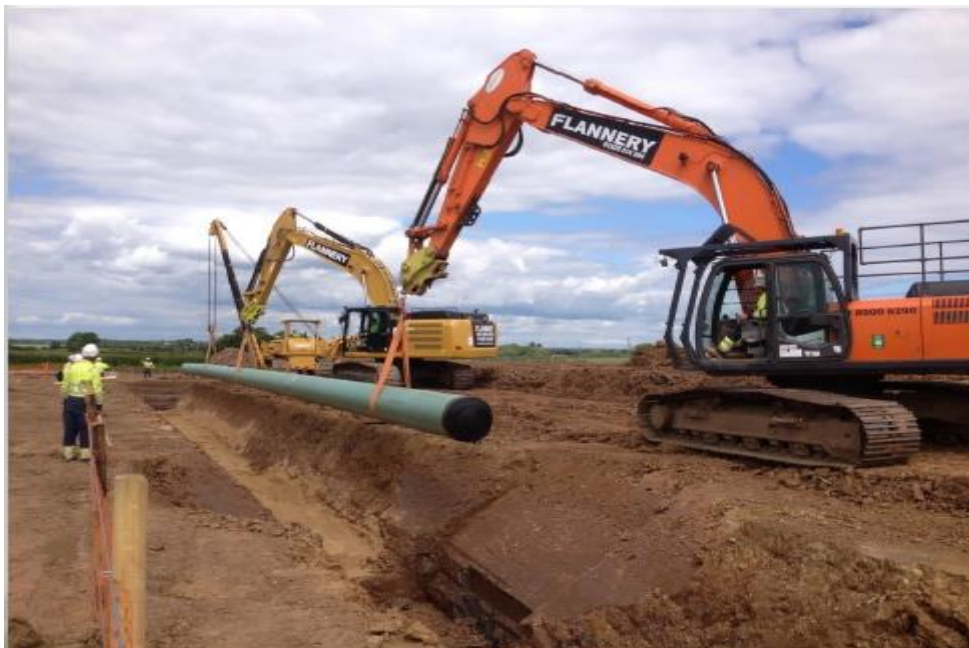
Figure 19: Diversion Works at Tall Trees and Morley Carr Farm Project
