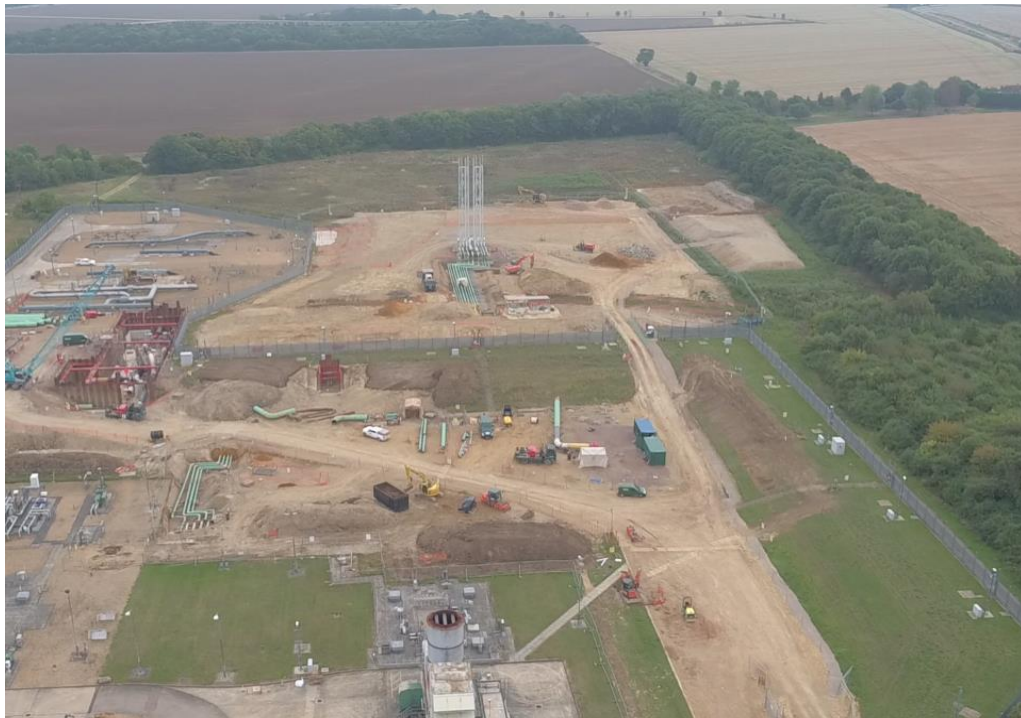
Figure 18: Aerial photo taken September 2016 mid-way through the Huntingdon Early Works delivery
