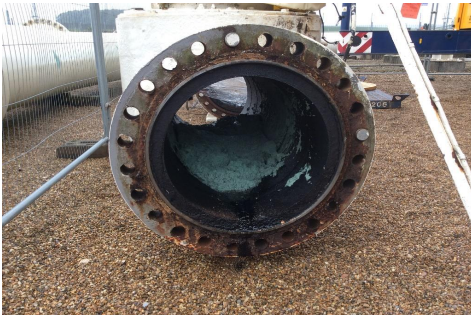
Figure 10: Feeder 2 valve removed from Bacton
