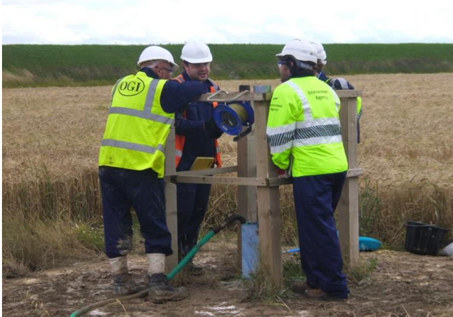
Figure 11: Environment Agency visit at Goxhill during the pump tests
