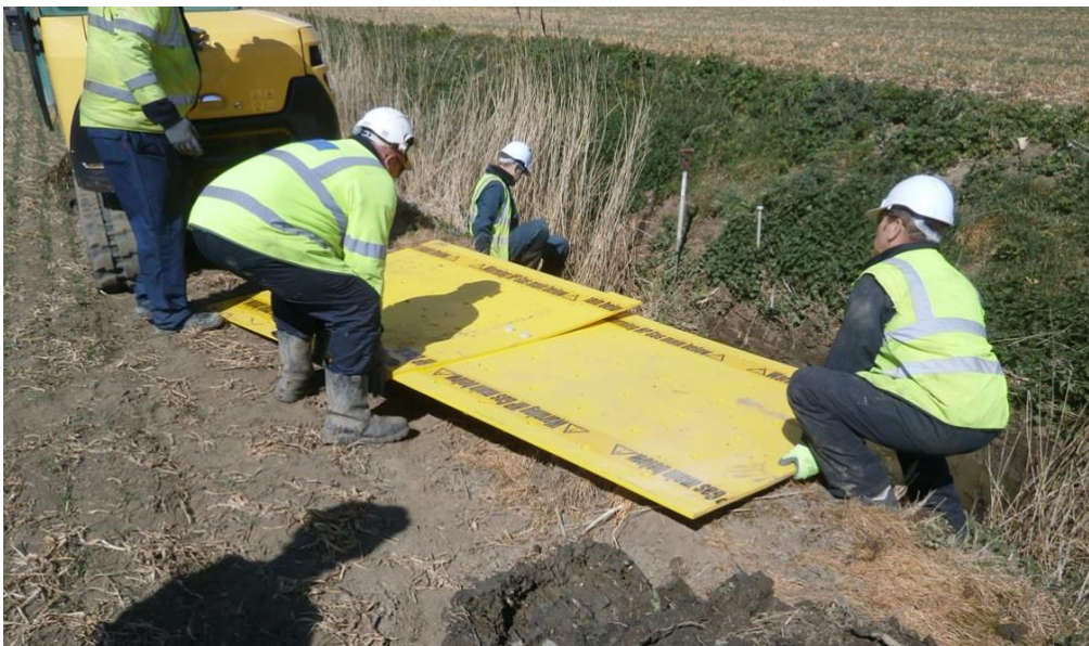
Figure 2: The installation of the new polyethylene pipe protection slabs
